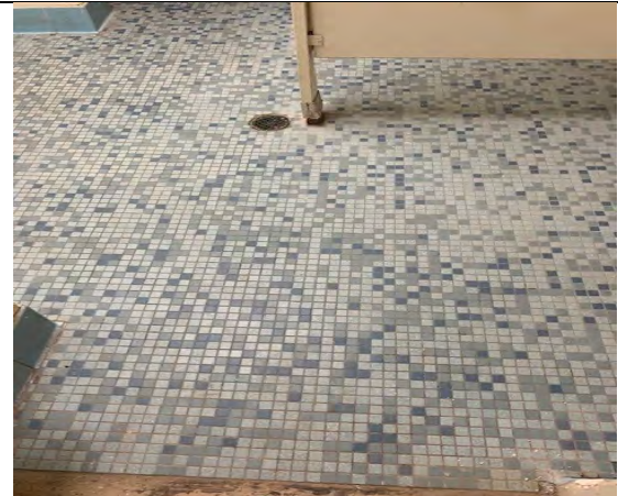
HM-10: 1" Blue Ceramic Floor Tile/Grout
