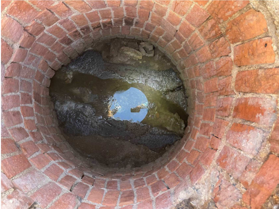
View within MH #42 to be rehabilitated.
