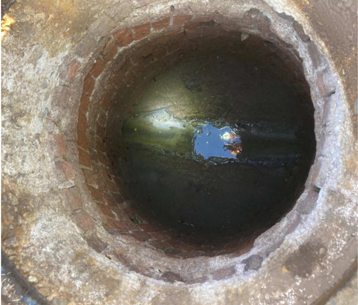
View within MH #58 to be rehabilitated.
