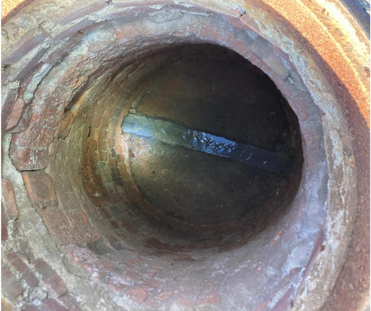
View within MH #60 to be rehabilitated.
