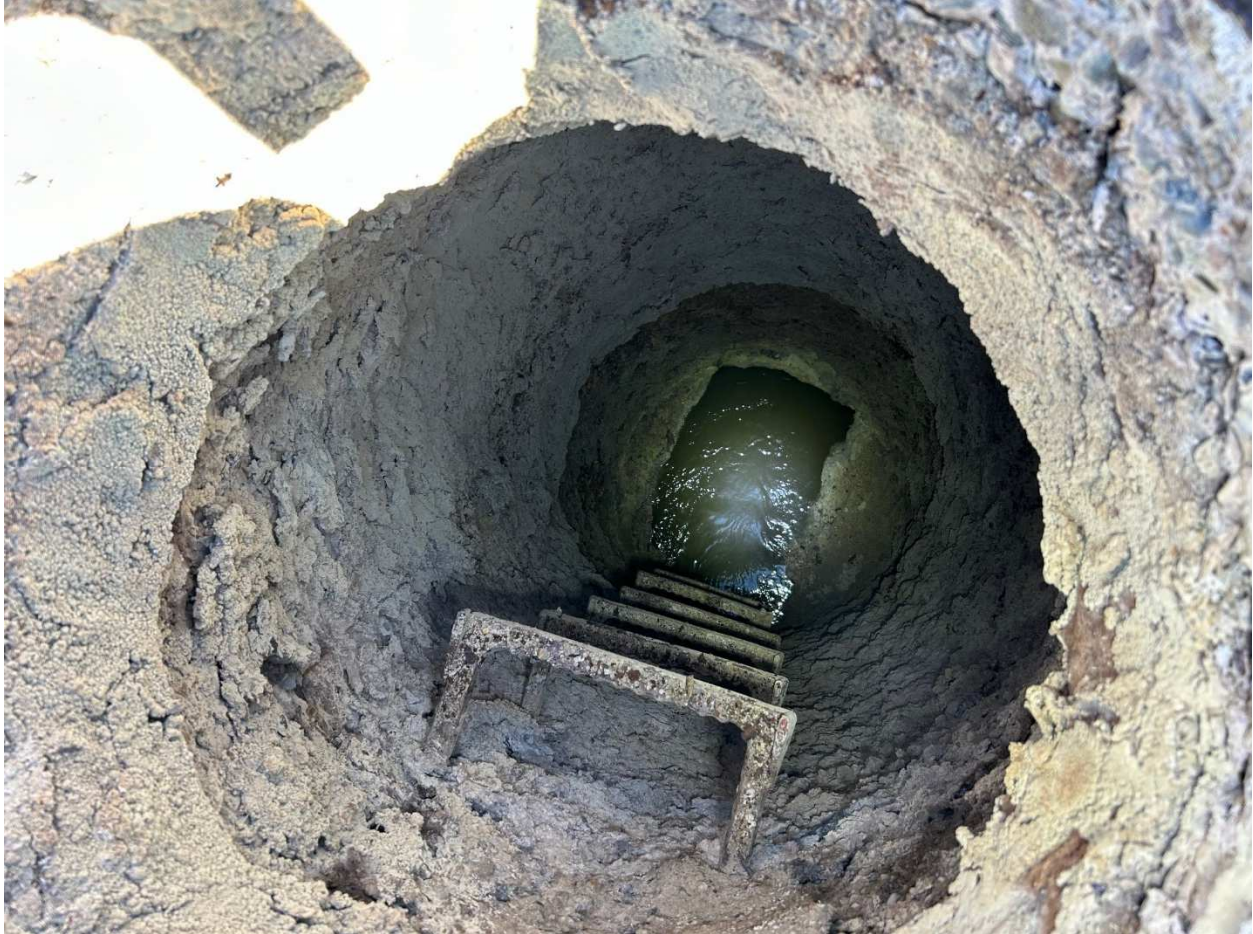
View within MH #1024 to be removed/replaced as a new 4' Diameter manhole.
