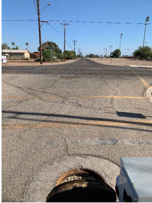
View north within B Street of MH No. 1102
