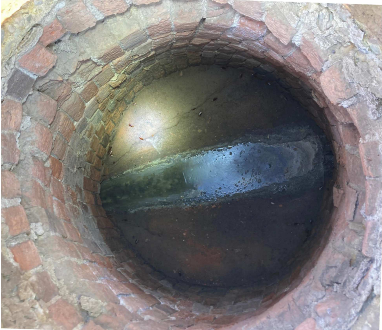
View within MH #55 to be rehabilitated.
