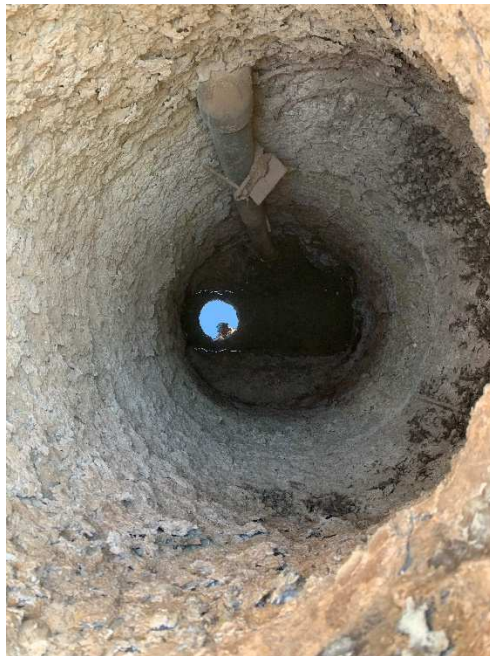
View within Manhole #1022 to be rehabilitated.
