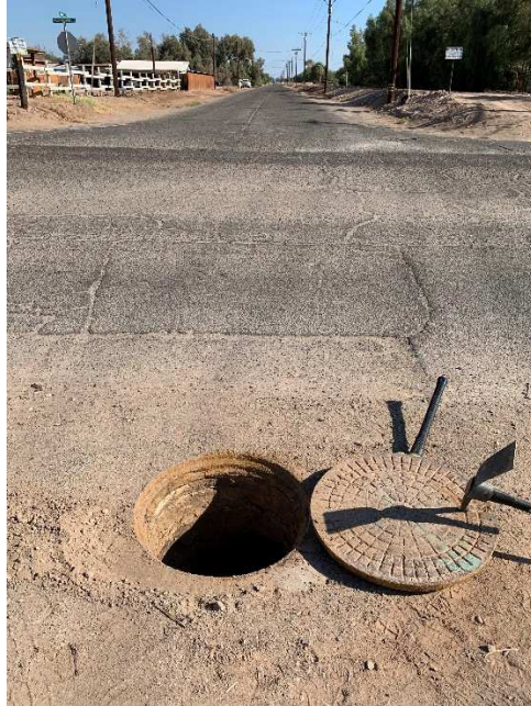
Manhole #1022 cover looking north.
