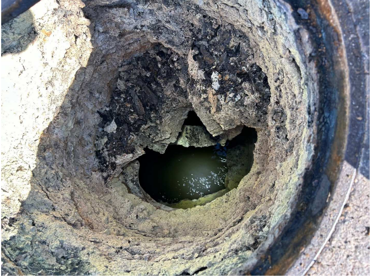
View within MH #348 to be rehabilitated.
