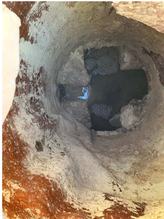
View within MH #1142 to be rehabilitated.
