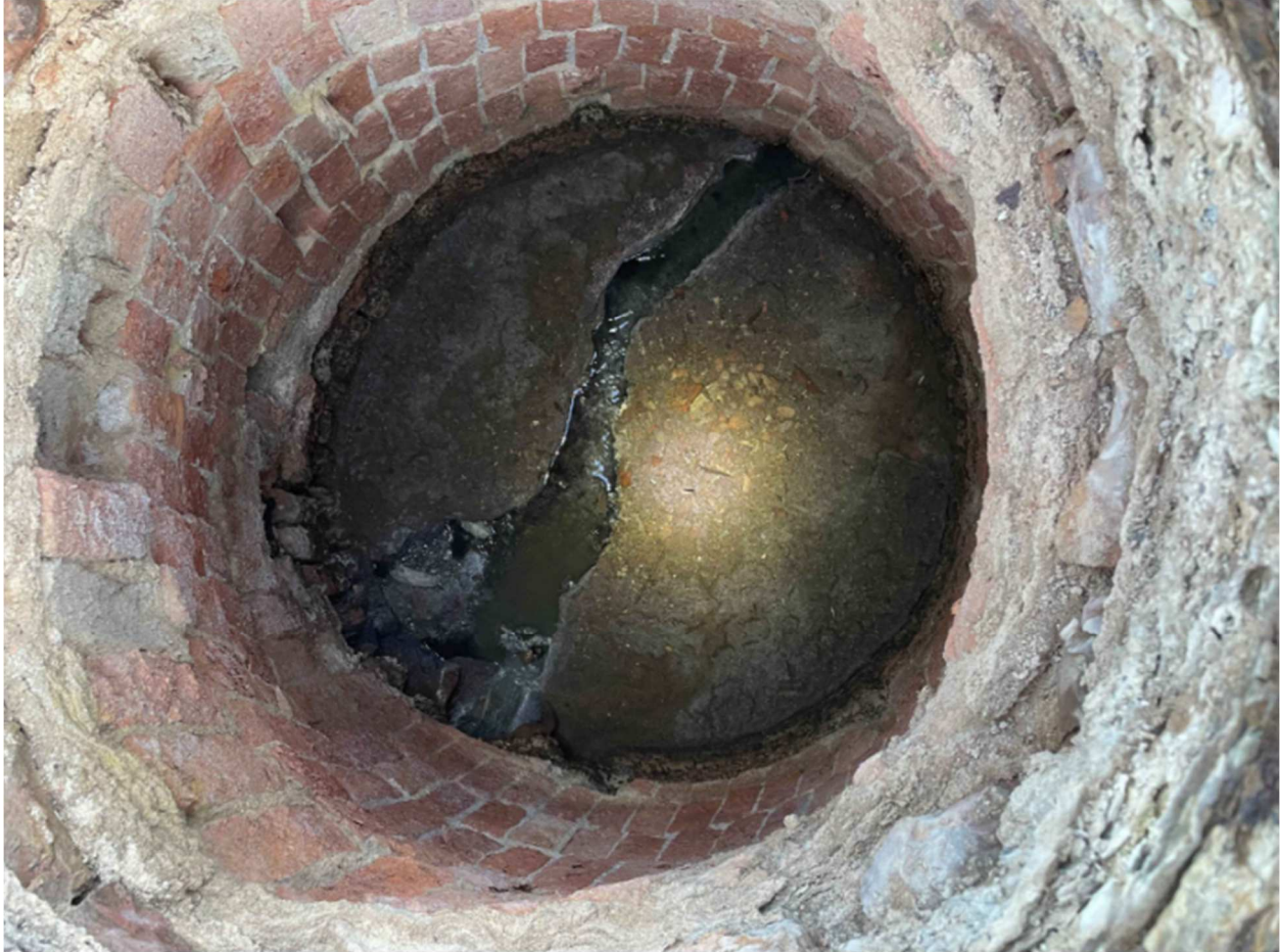
View within MH #51 to be rehabilitated.
