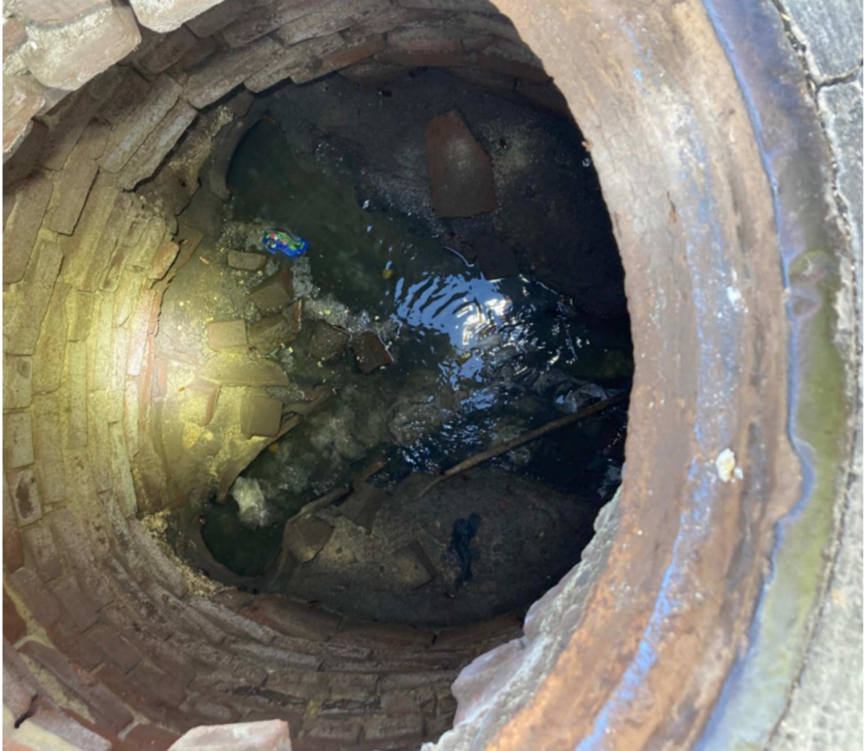
View within MH #54 to be rehabilitated.
