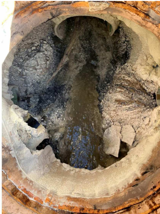
View within MH #359 to be removed and replaced with a 6' diameter manhole per Detail No. 1 on Sheet No. 3 of the bid set plans.
