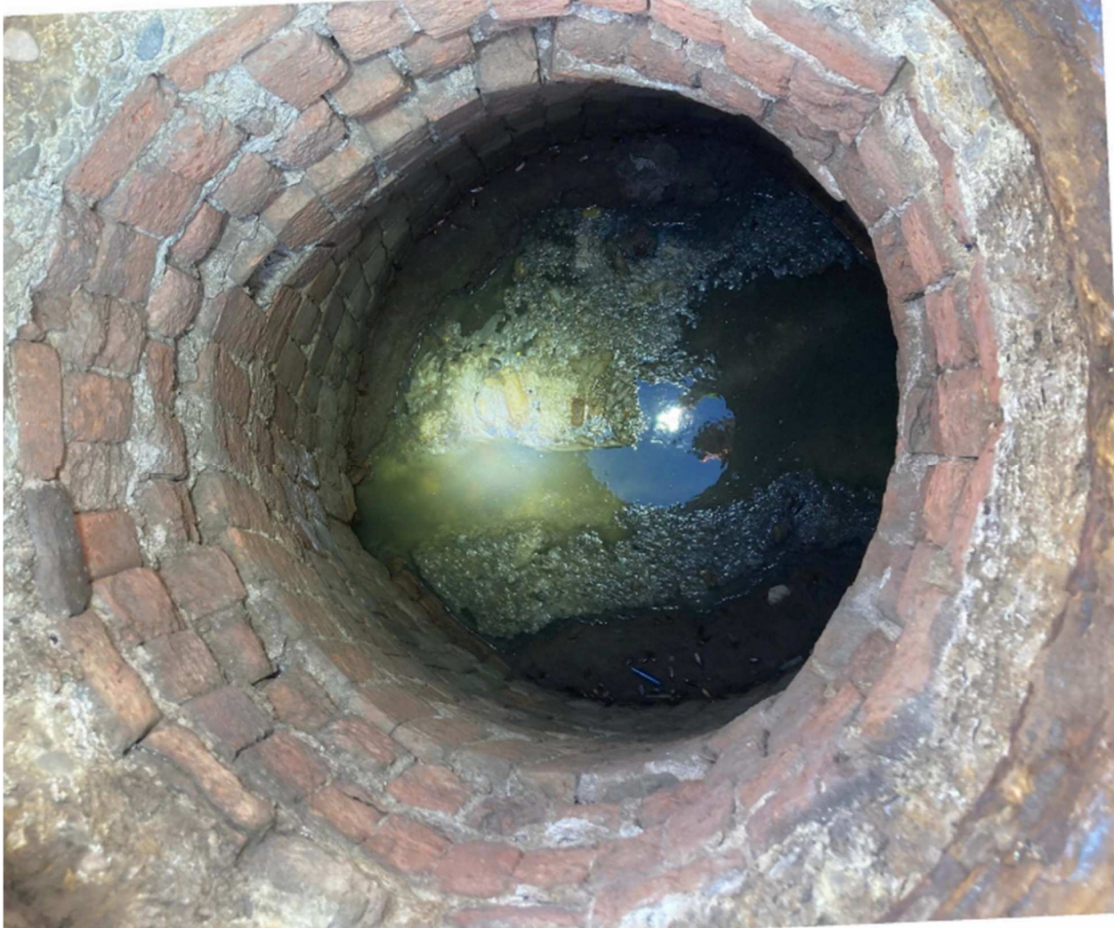
View within MH #56 to be rehabilitated.
