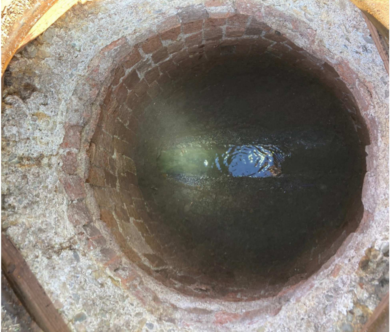
View within MH #59 to be rehabilitated.
