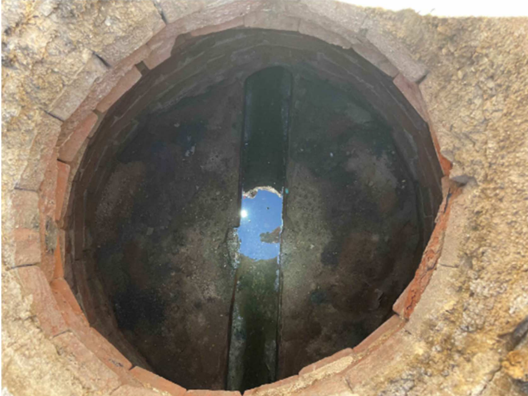
View within MH #28 to be rehabilitated.
